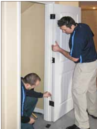
New doors and hardware are installed.
